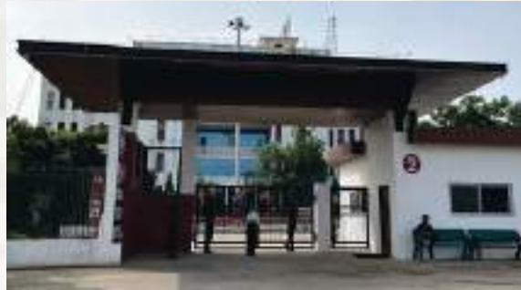
Major Facelift of Main Entrance Gate (Gate No 2).
