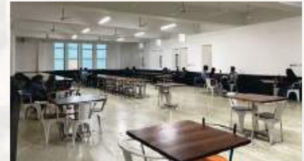
Renovation of Students' Canteen
